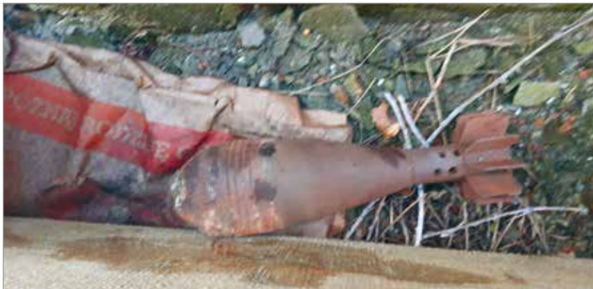
Second World War mortar shell, found during the roof renovation
